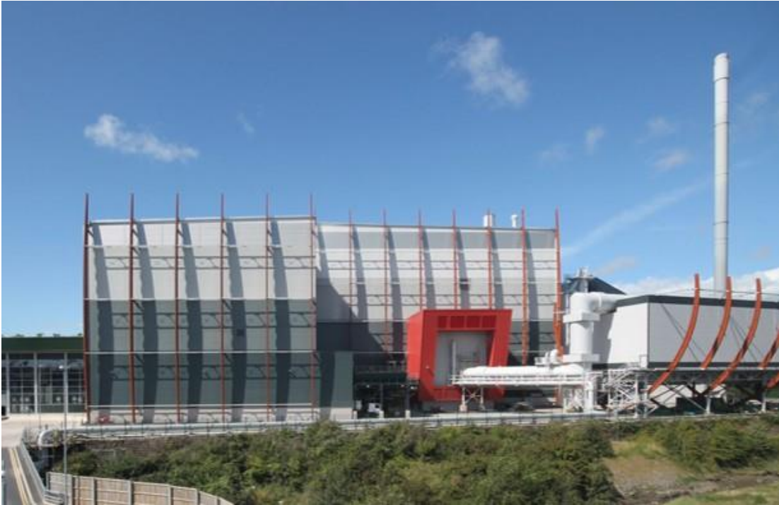
Plate 1-2 Indicative image of a typical EfW facility (North Yard, Devonport, Plymouth)
